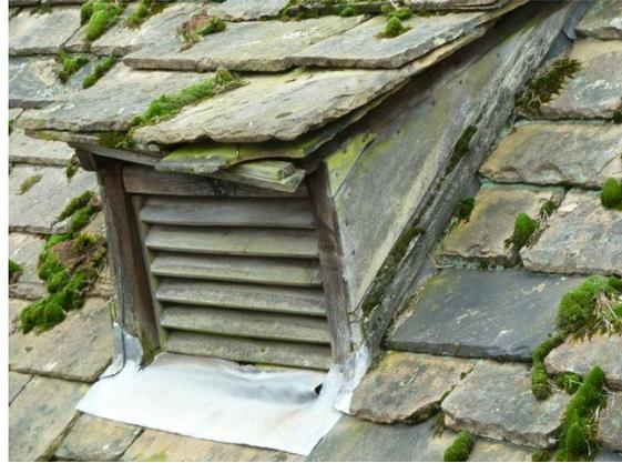
The mill before works had significant roofing issues, with many rafters either bowed or cracked and a very clear undulation in the main roof slope. The main frame had shifted and was misaligned with the stonework below. Most stone slates were salvaged and best conservation principles followed.
