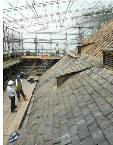
The stone slates were stripped, numbered and stored whilst structural repairs were undertaken. They were then replaced in their original positions using new oak pegs. Finally lime 'torching' was used internally to weatherproof the roof.
